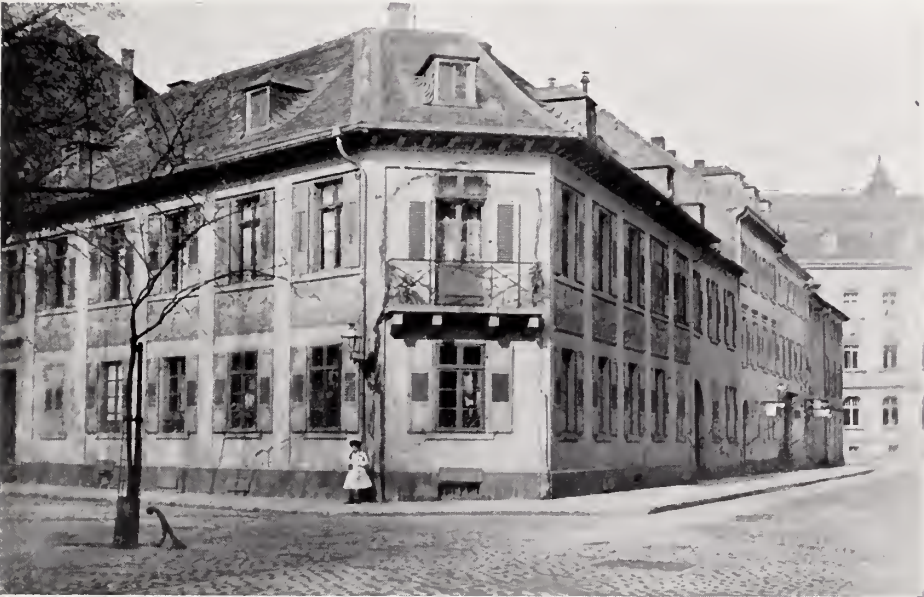
Illus. 198a.—Karlsruhe, showing successful treatment of acute-angled corner on the Luöwzig Platz. See Fold Map IV. and Illus. 114a.
